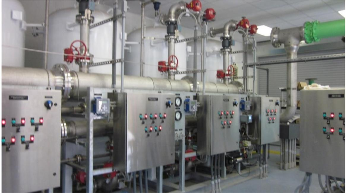
***A Nitrate Removal Ion Exchange Treatment System***
