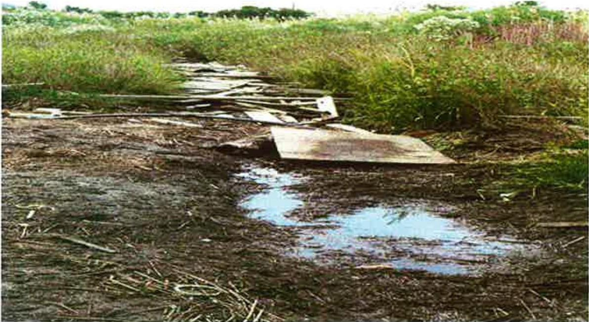
This floodwater ditch, filled with sand and debris, is in need of maintenance to prevent mosquito breeding.
