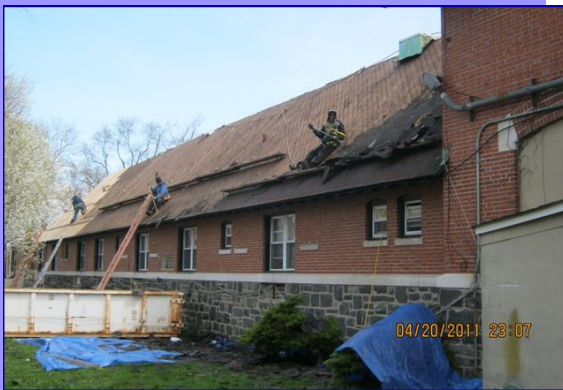
Jones Manor renovation
