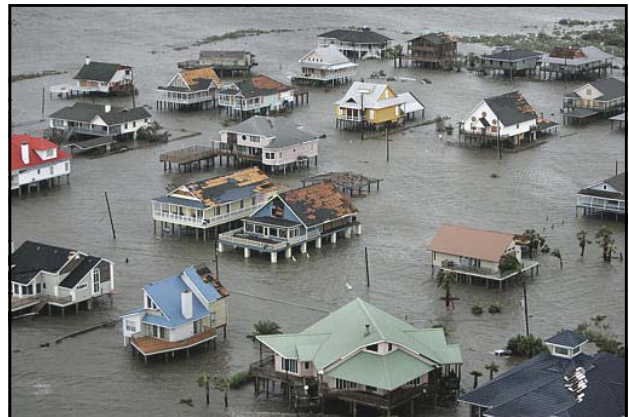
Elevated homes in Sweet Lake, LA (near Lake Charles) after Hurricane Rita (09/24/05).
