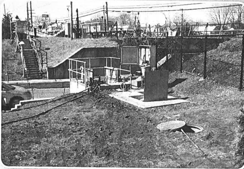
Reconstructed wet well/relocated electrical equipment
