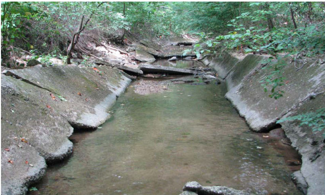
Photograph of existing deteriorated concrete trapezoidal channel
