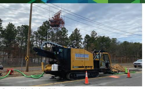
Eastern Utilities Services (EUS) specializes in directional drilling and trenchless technology. Utilizing production style directional drilling, EUS safely installs the maximum amount of footage possible by using an advanced mud management system and specialized equipment, including a state-of-the-art reclaiming system, yielding boring rates of up to three times greater than its competitors.
