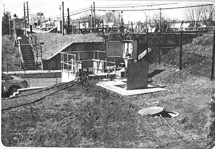
Reconstructed wet well/relocated electrical equipment
