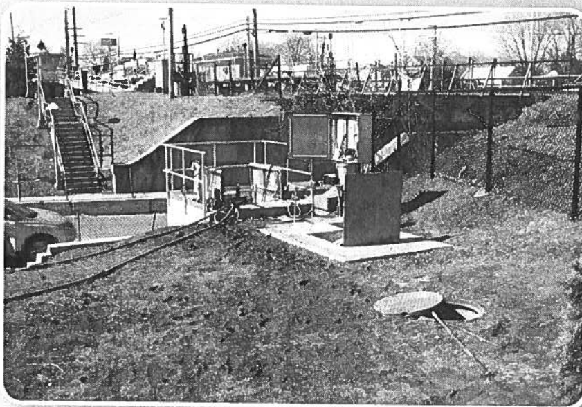
Reconstructed wet well/relocated electrical equipment
