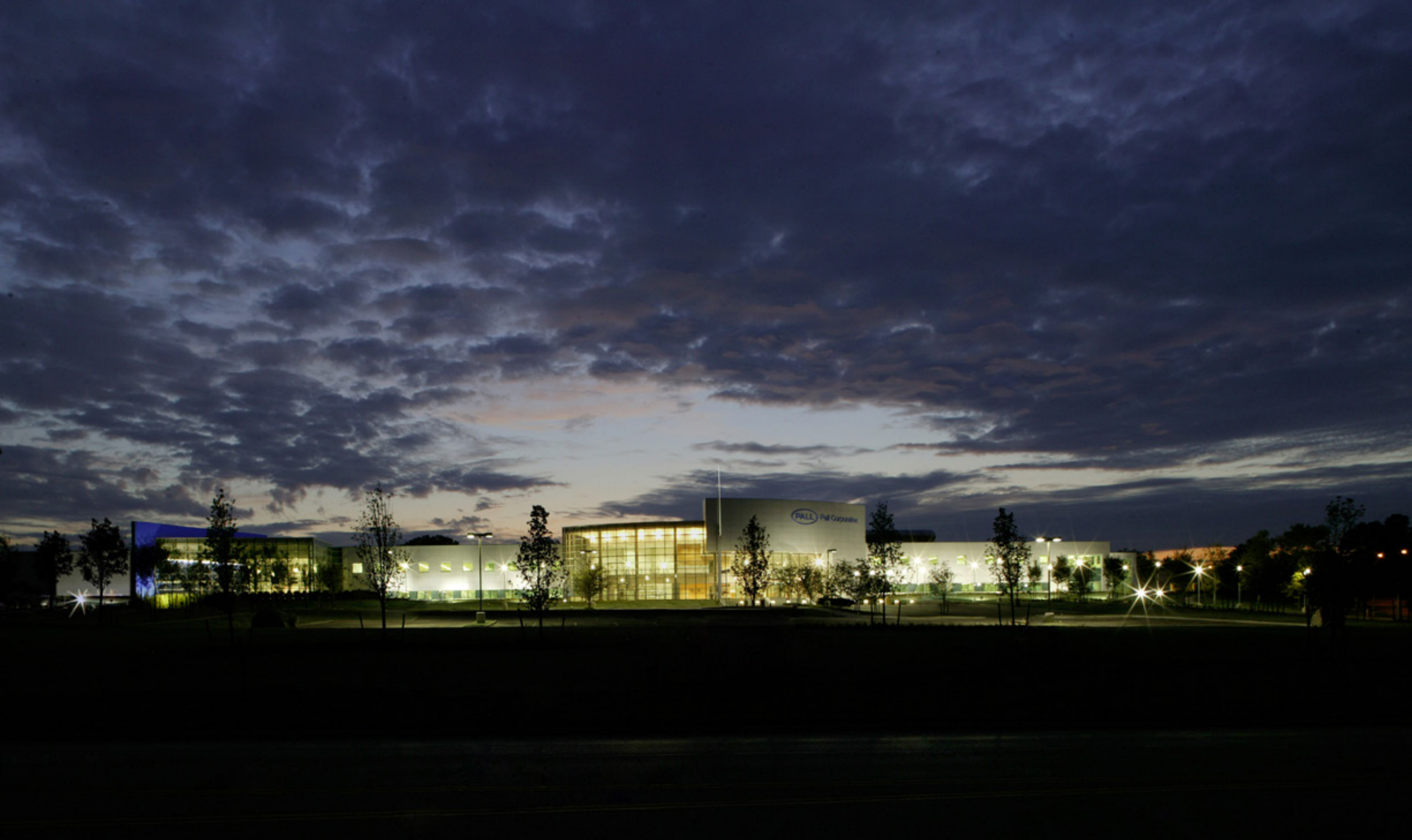
PALL CORPORATION CORPORATE HEADQUARTERS | Port Washington, New York
