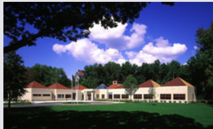
Kings Point Village Hall and Police Station Kings Point, New York
