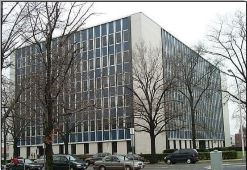
(View of County Clerk's Office Building - 240 Old Country Rd, Mineola, New York)
