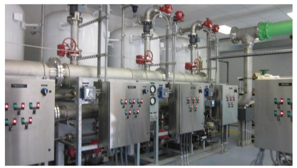
A Nitrate Removal Ion Exchange Treatment System
