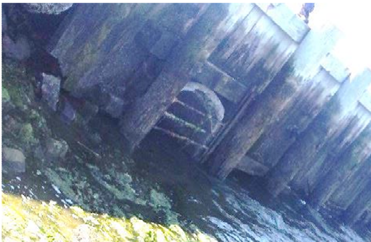
Figure 8: Bayswater Boulevard Outfall
