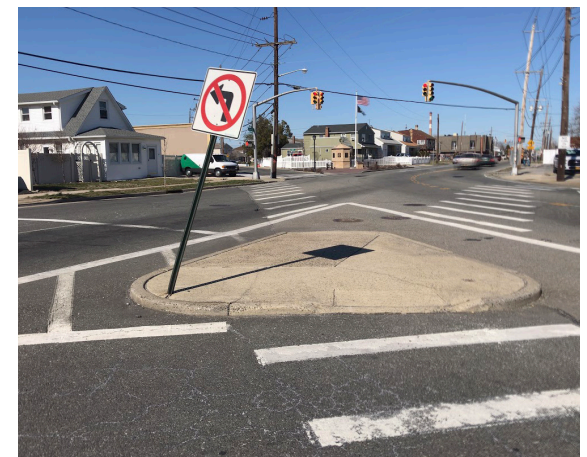
Figure 4. North End of Long Beach Road
