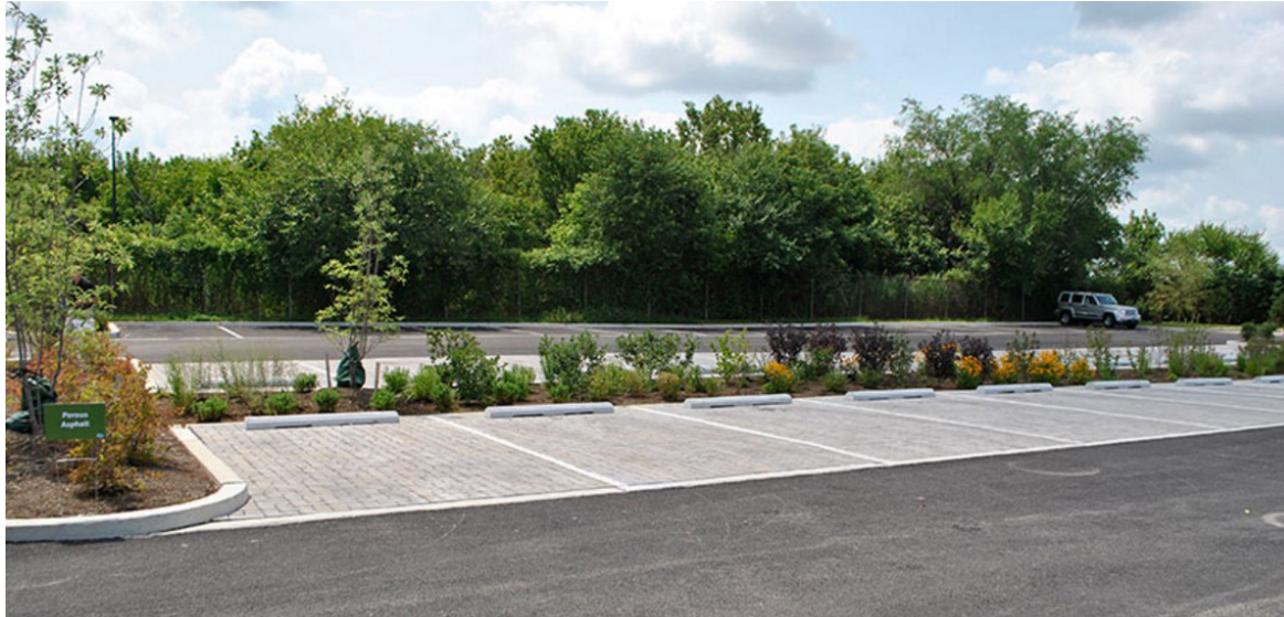
Bioswales (Photo Credit: Philadelphia Water Stormwater Management Guidance Manual)
