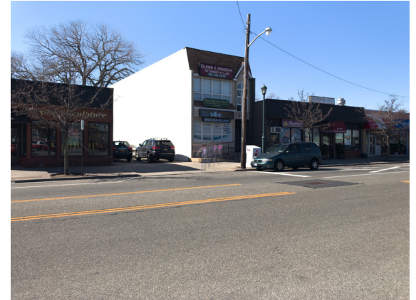
Existing Retail Along Long Beach Road
