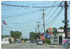
Pedestrian safety improvements are needed along Grand Avenue.
