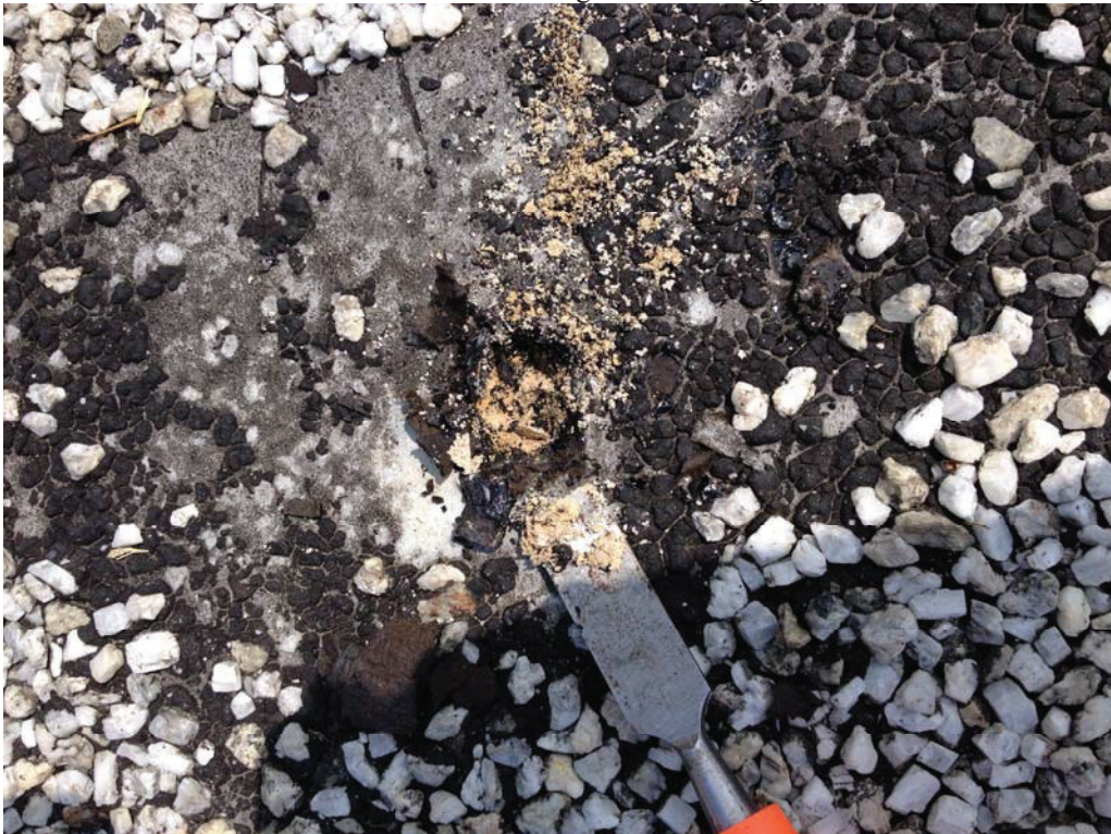
Asbestos Containing Roofing Material (all layers)
