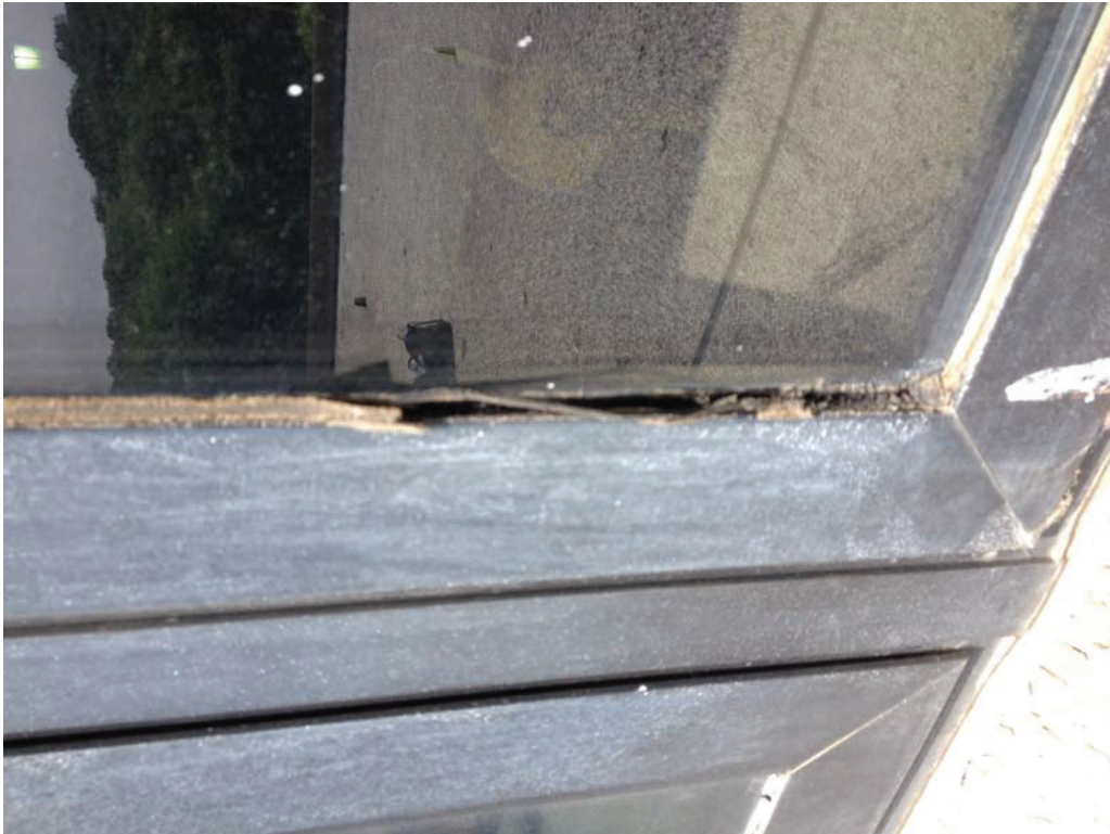
Asbestos Containing Window Caulk
