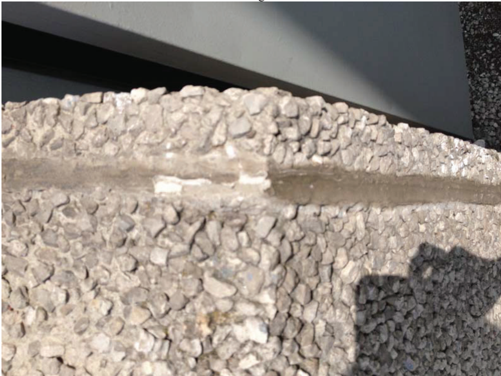
Non-asbestos containing building caulk (expansion joint)
