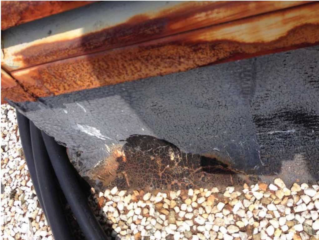
Asbestos Containing Roof Flashing.
