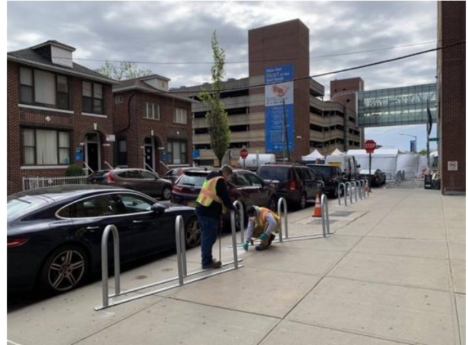
Bicycle parking being installed near a hospital in Elmhurst, Queens. https://twitter.com/NYC_DOT/status/1258433264731242498?s=19
