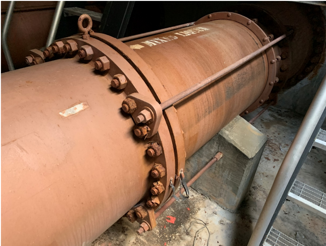
North FST Distribution: Non-LBP Red Pipe Paint
