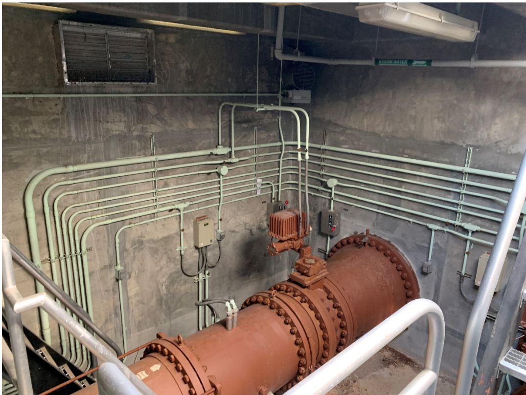
North FST Distribution: Non-LBP Gray Conduit Paint
