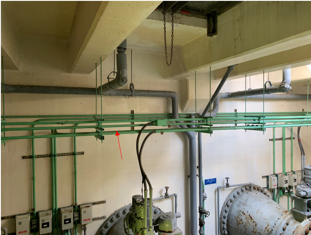
South Distribution: Non-LBP Green Paint on metal conduit
