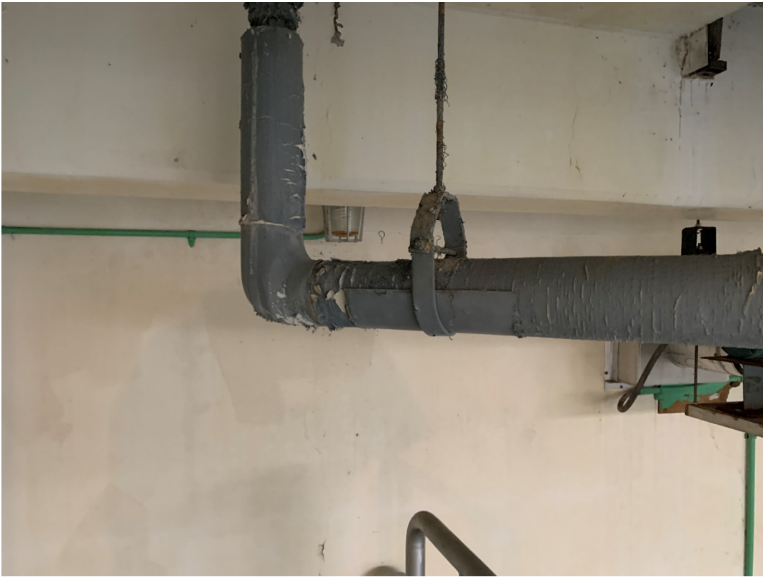
South Distribution Tanks: Non-ACM Mud Joint Packing
