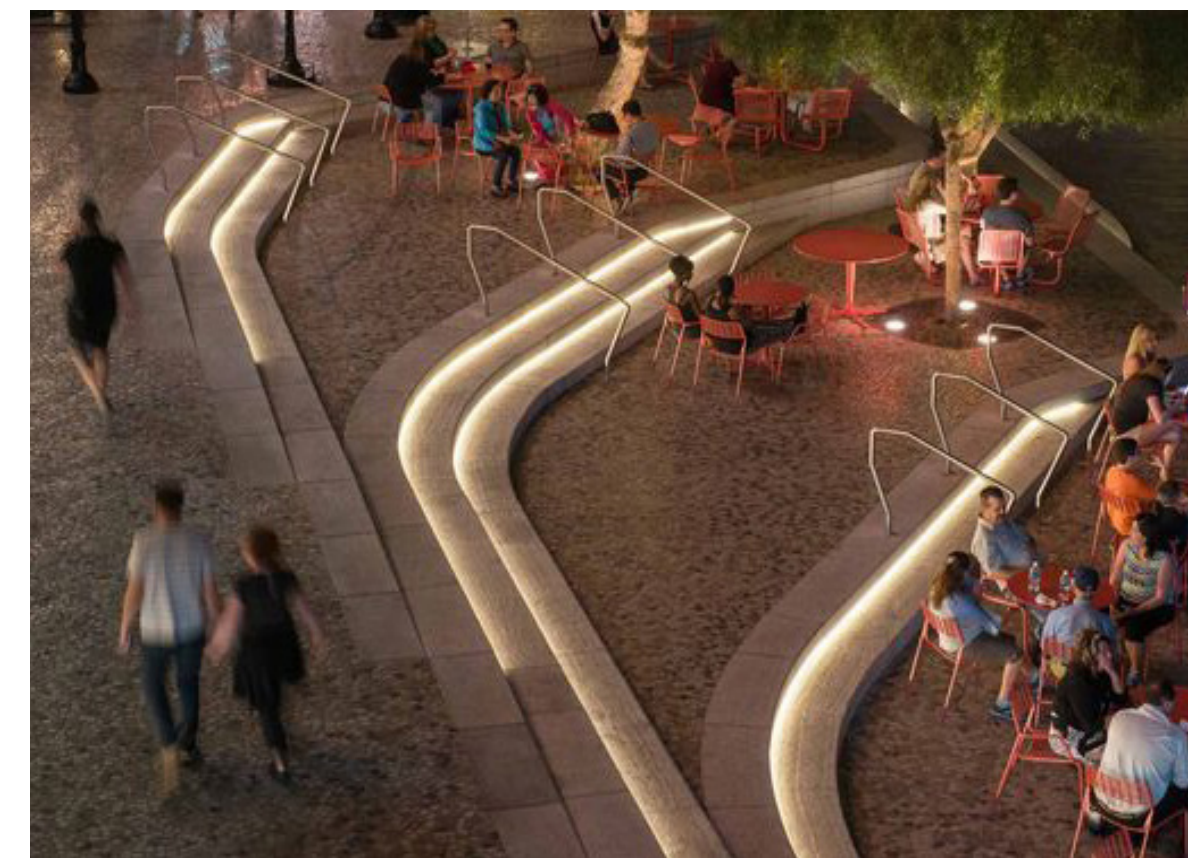
TYPE TXN LINEAR TAPE LIGHT AT STEPPED SEATING
