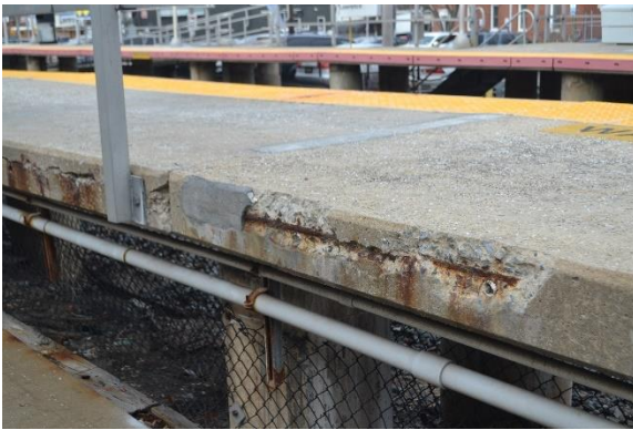
Lawrence LIRR Station Platform
