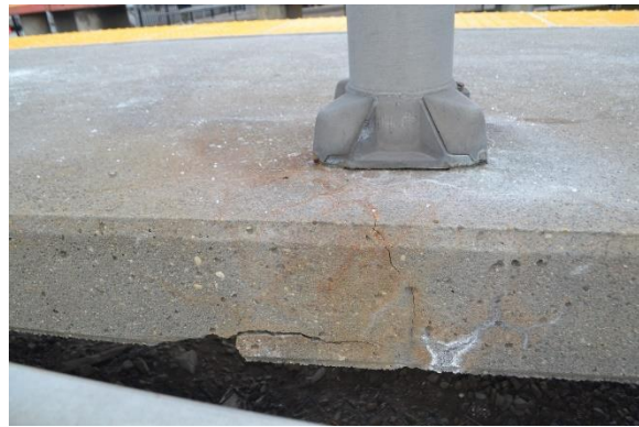
Inwood LIRR Station Platform
