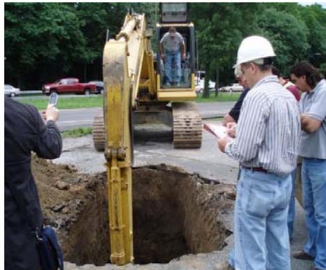
*Public Health Engineer Salvatore Caruso Inspects a Test Hole for a Commercial Sewage Disposal System in Glen Head*
